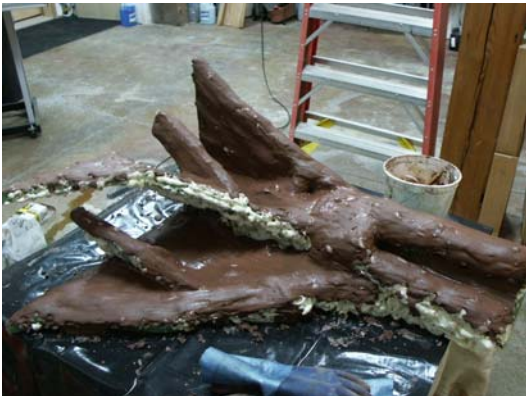
Mortar partially applied. It helps to lay the piece on the side to let gravity work for you.
